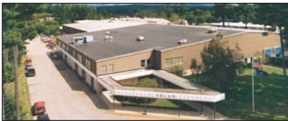
WILLISTON, VT, U.S.A. - Velan Valve Corp. 155,000 sq. ft. (14,400 m 2 ) 2–24" (50–600 mm) forged & cast steel gate, globe and check valves - VELNORTH 8,000 sq. ft. (743 m 2 )
