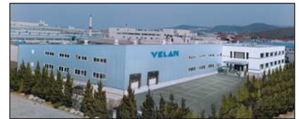
ANSAN CITY, SOUTH KOREA Plant 2 65,000 sq. ft. (5,800 m 2 ), 2–12" (50–300 mm) cast steel gate, globe, check, ball and knife gate valves
