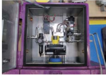
K-Cab 阀门控制单元防火箱 K-Cabhousing control set protection
