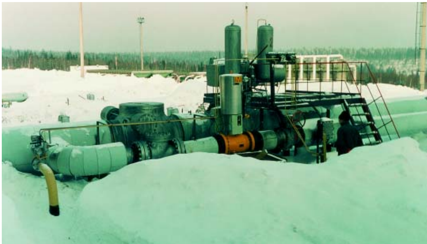
flowline shut-off valves gas production plant, N/E Netherlands (by courtesy of NAM)
