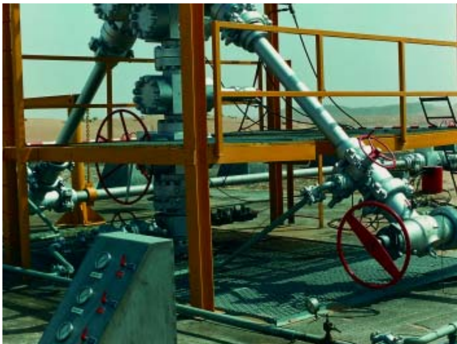
adjustable choke valves 7 1 / 16 " API 10,000 with inconel cladding, gas production field UAE
