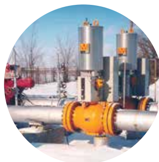
16" / ASME 600 Axial Control Valve
