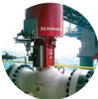
24" / ASME 1500 Axial Control Valve
