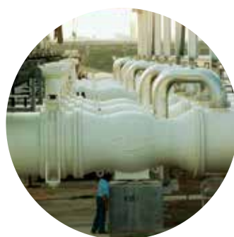
72" / ASME 175 Axial Check Valve
