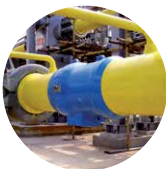
20" / ASME 2500 Axial Check Valve
