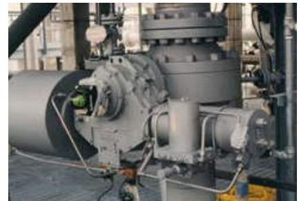
This 12-inch ASME 300 Class valve was used for Vinyl Chloride Monomer (VCM) furnace isolation operating at 1200 F (650 C) with 120 psi (8 bar).
