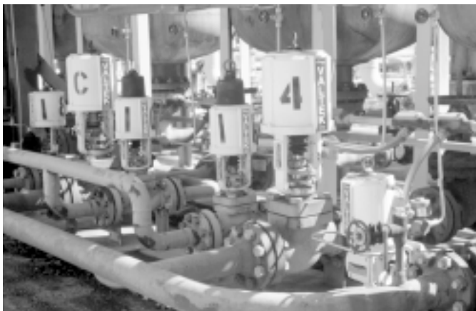
This cryogenic Mark One is used for aerospace testing as an O 2 vent valve.
