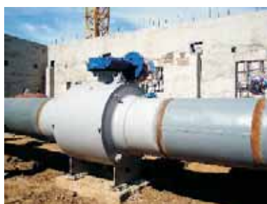
全焊接球阀正在中俄原油漠大线安装 Fully welded body ball valve under installation at Sino-Russia Crude Oil Project Mo-Da Line
